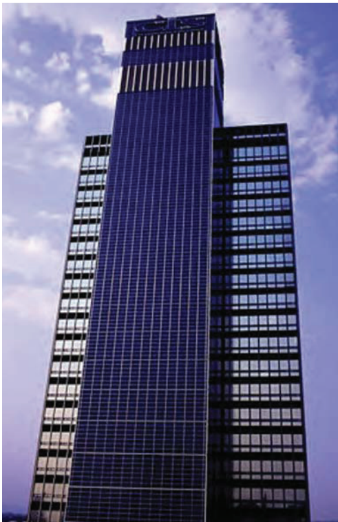
The CIS Tower, Miller Street, Manchester, with PV solar panels
